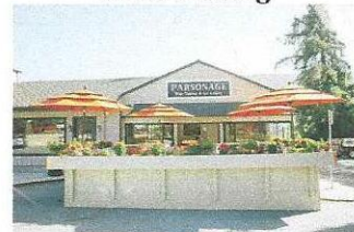
January 30 th at Parsonage Winery Carmel Valley Village
